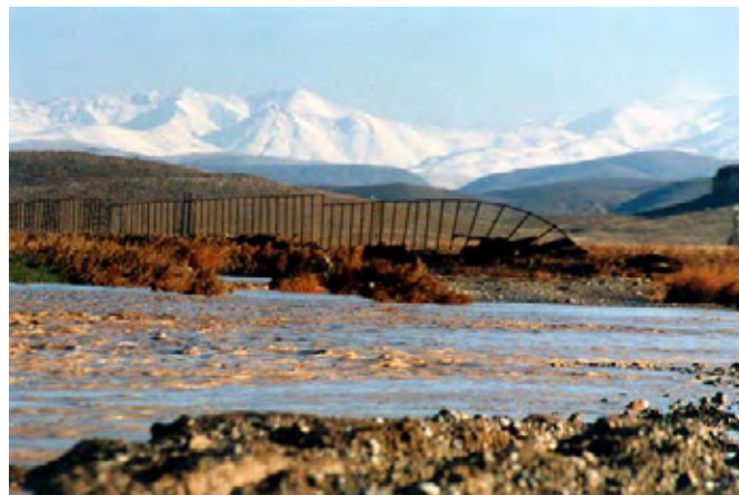
Floods destroying sections of the metallic enclosure of Pasargadae
