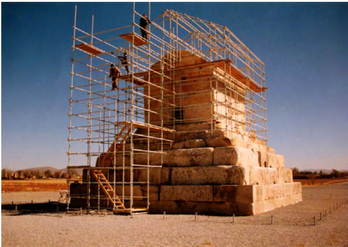
Mausoleum of Cyrus the Great, building scaffoldings
